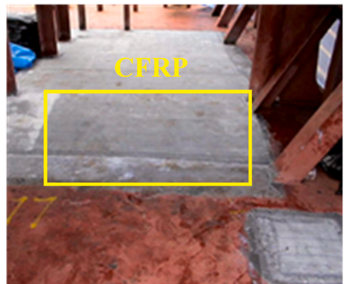
Fig. 2. Repairing corroded deck on FOU with CFRP.
